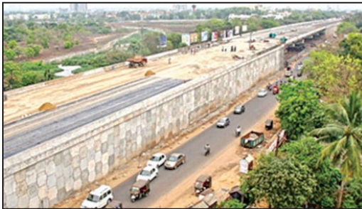
FIGURE 7: A grade separator Under Construction
