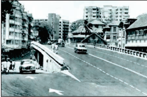
FIGURE 6: Kemps Corner Flyover, Mumbai
